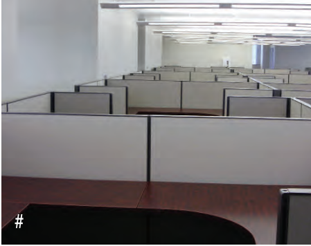
Panel runs should be installed straight and parallel to each other.
